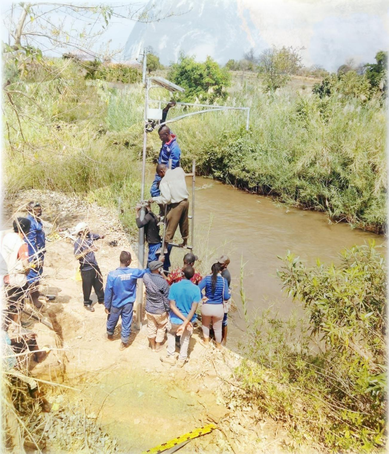
*Installation of Telemetric station-an early warning system in Malawi*
